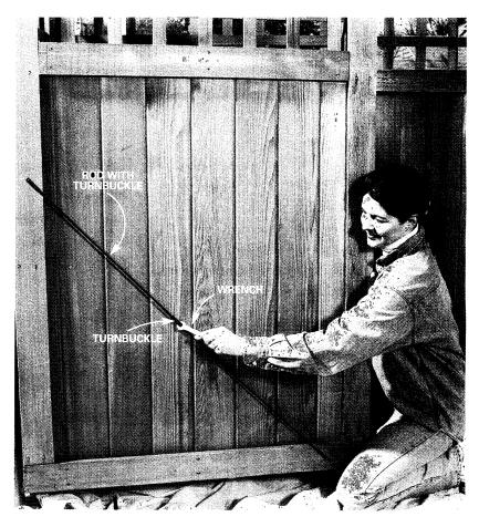
REALIGN sagging gates with a turnbuckle.
